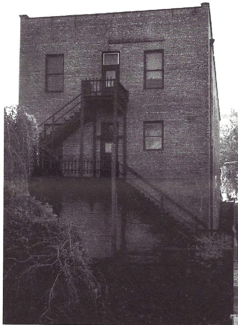
The south side of Pioneer Hall with newly repaired and reconfigured stairway
